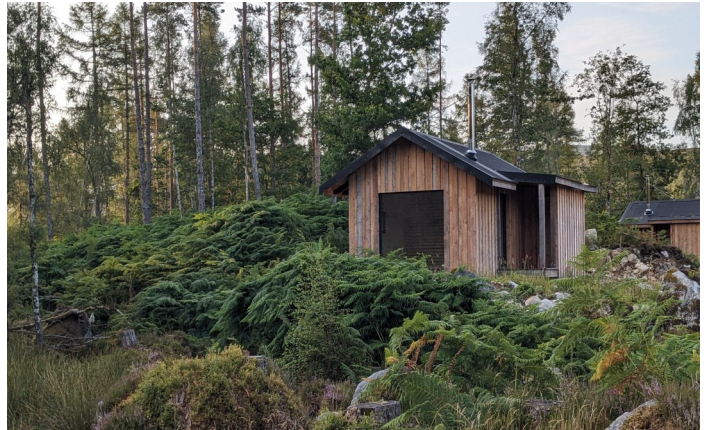
Our cabins fully clad and watertight for the winter
