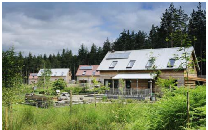
Catoe Brown's award winning affordable housing development at Ardgael (pictured above) is a good precedent for our project at Ardochy
