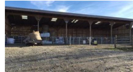
General Purpose shed at Greenfield.
